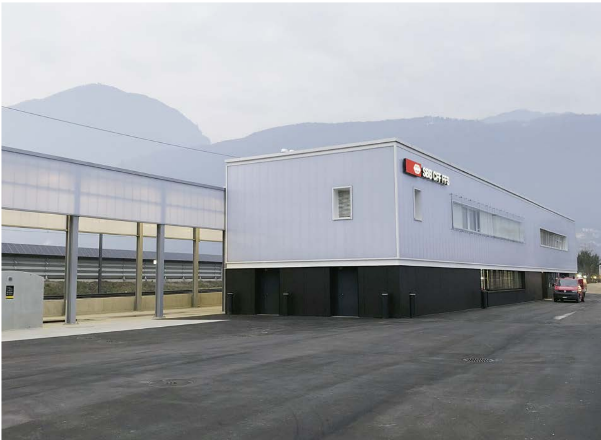
NEAT, Interventionszentrum Melide.
