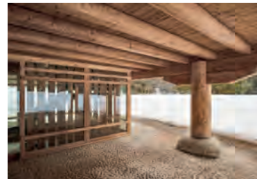
6 Der traditionelle Holzbau blieb erhalten. | The traditional wooden construction has been preserved.
