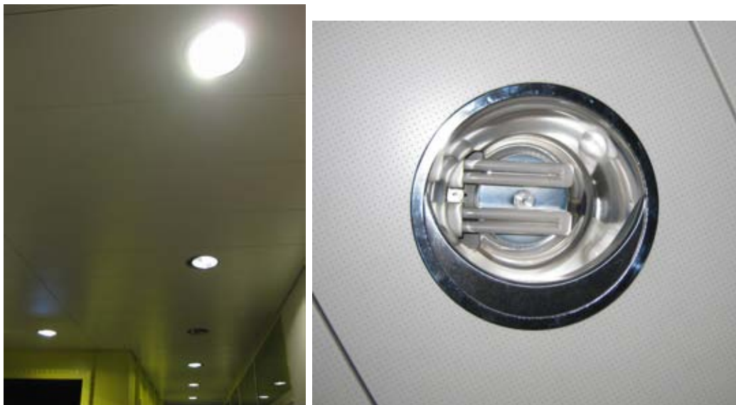
(a) Ceiling with recessed lighting (b) Close-up of recessed bulb holder with metallic-reflective surface
